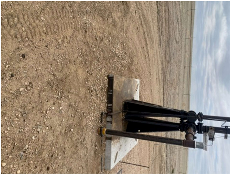
STAINED SOIL REMOVED/FLARE REPAIRED AND CLEANED
