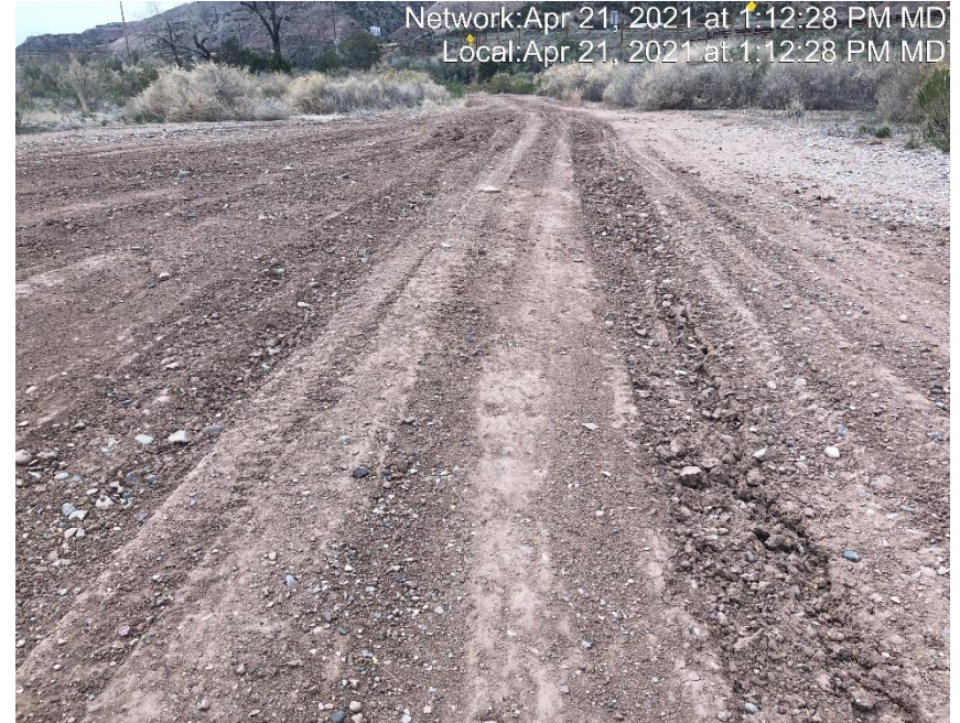
Photo #3579 location lacks stabilization.
