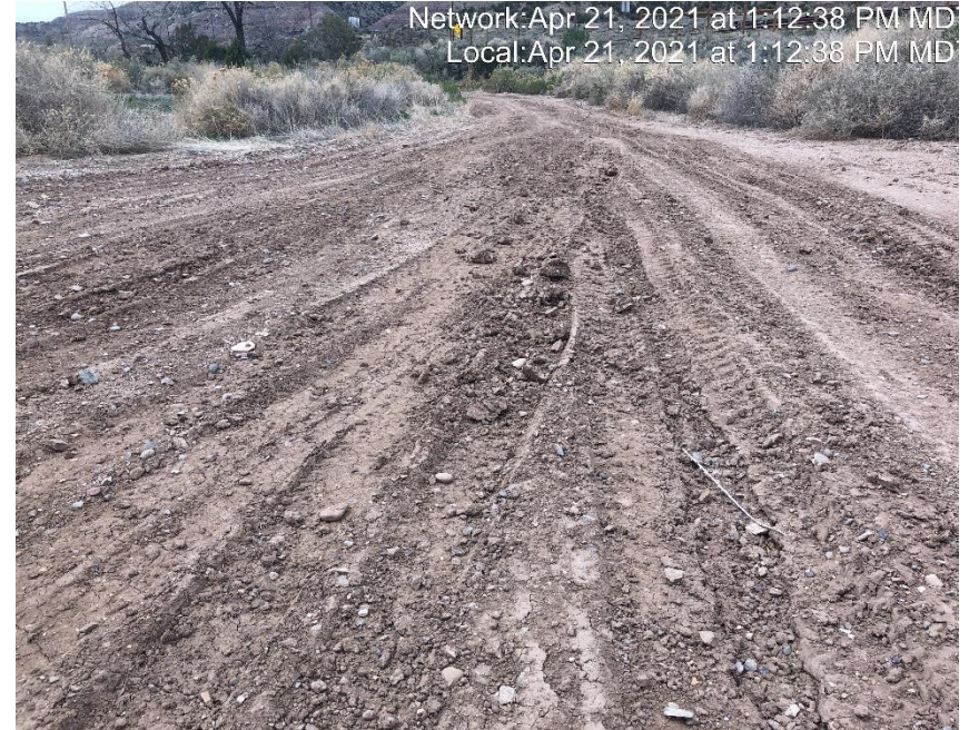
Photo #3580 No form of tracking BMP at entrance to location.
