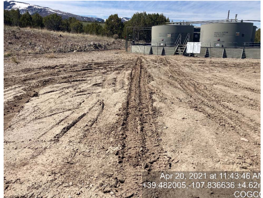
Lack of stabilization/compaction
