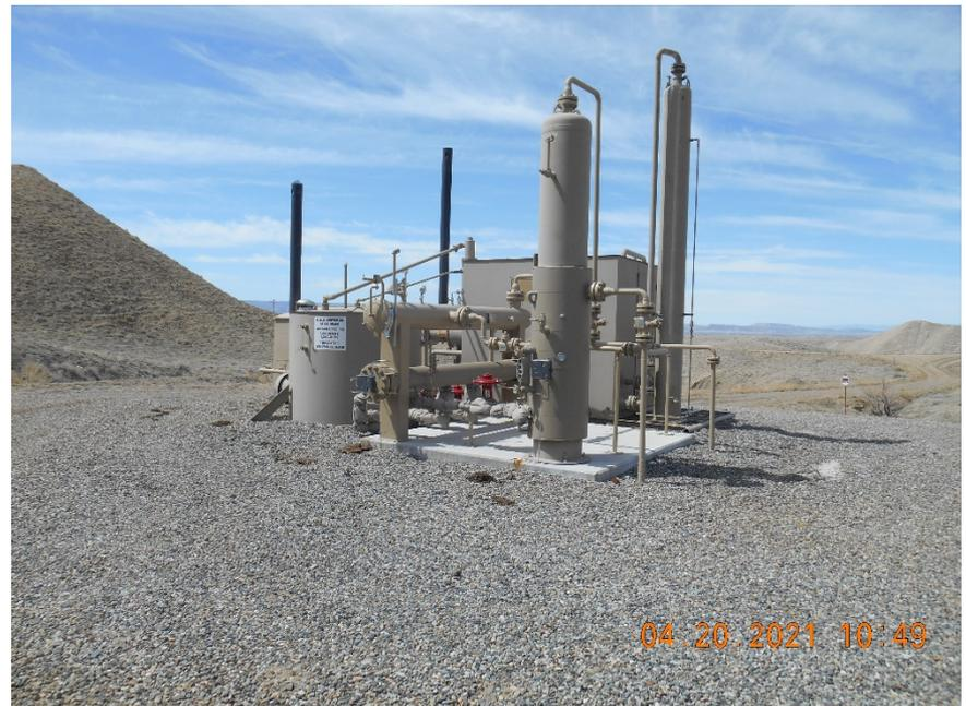
**Separator, Dehydrator, Meter housing and Tank**
