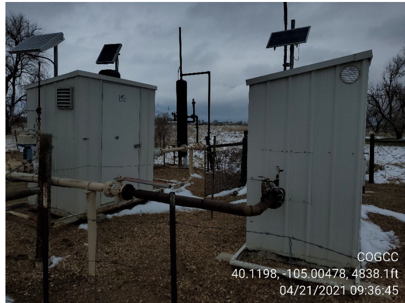
Photo 6 Jillson A Tank Battery meter house; KPK Jillson meter on left; presumed Crestone Jillson A meter on right
