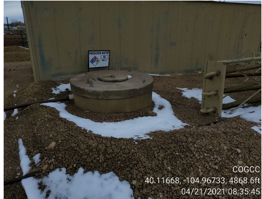
Photo 2: Buried concrete produced water vessel on east side of compressor building.
