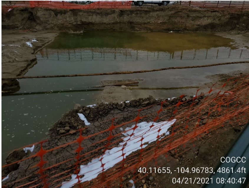
Photo 11: Groundwater in eastern excavation.
