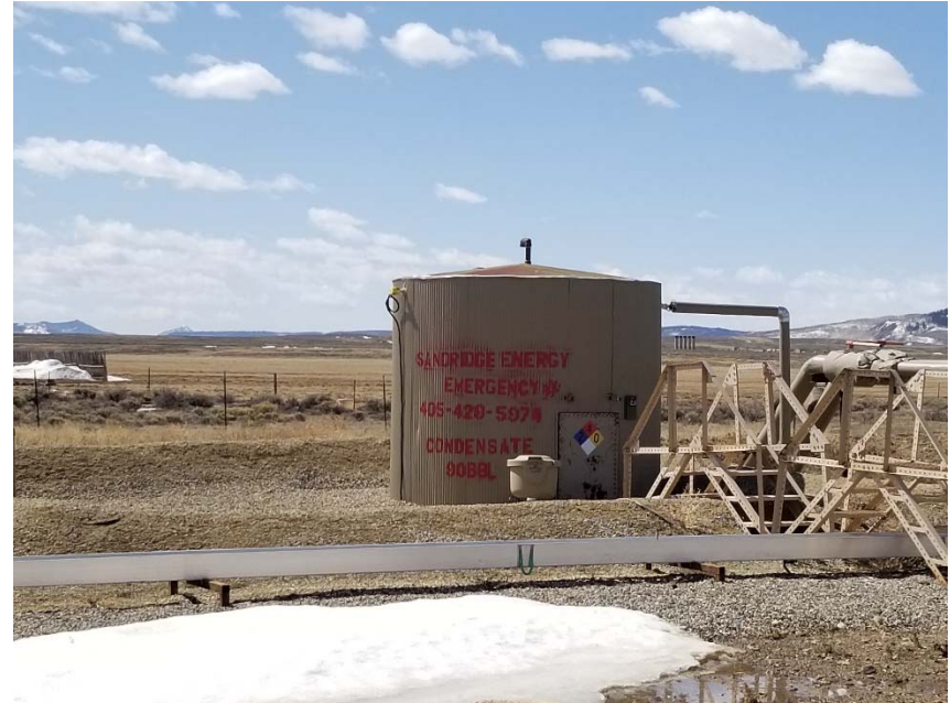
Photo 8. Tank label incomplete/inaccurate.
