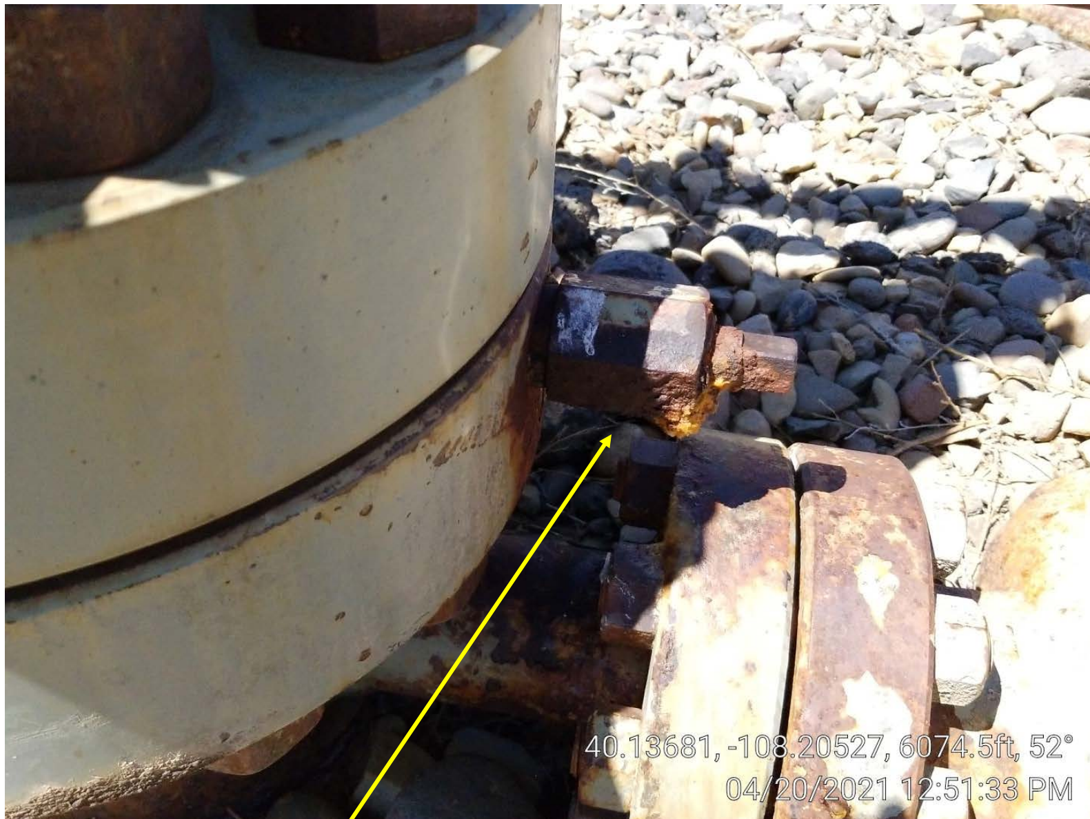
Photo 3. Well gas leak.
