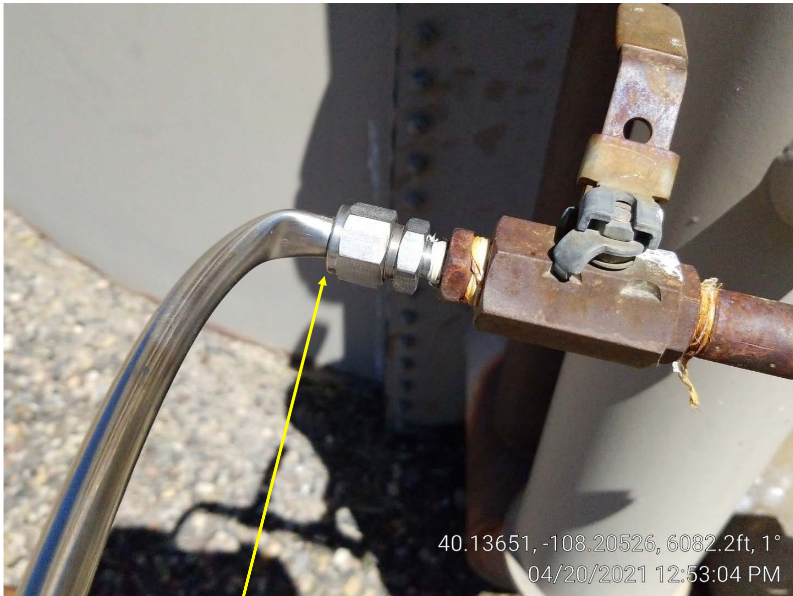
Photo 6. Gas leak at tank.
