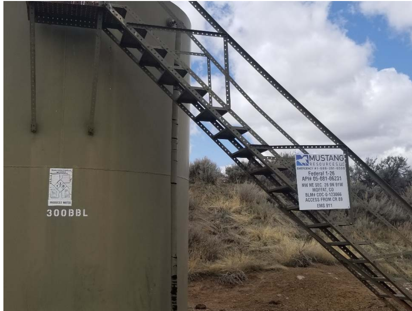
Photo 2. Battery sign incomplete/inaccurate. Tank label incomplete/inaccurate.
