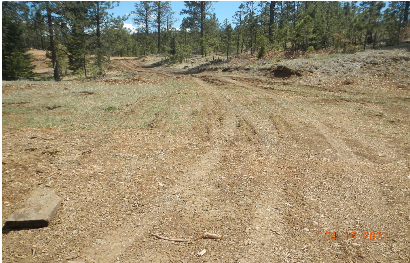
Photo 4. There was a road built to the south of the location. The road is causing disturbance of the interim reclamation. Vehicle access needs to be prevented.
