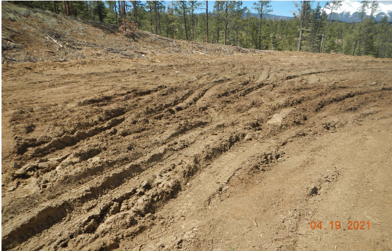
Photo 5. There is vehicle rutting and disturbance that occurred which needs to be repaired and reclaimed.
