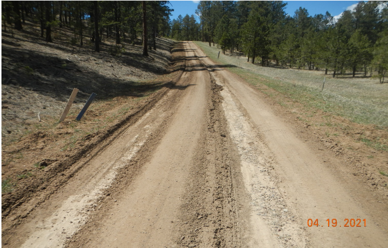
Photo 1. There was vehicle rutting along areas of the main road coming from wet canyon. Areas of rutting need to be maintained and stabilized.
