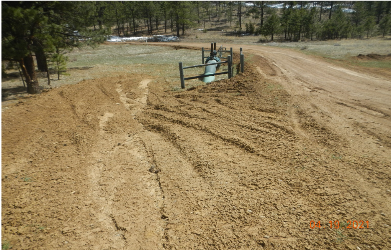
Photo 3. Facing southeast along the access road There is grading disturbance which needs to be reclaimed near the pig launcher.
