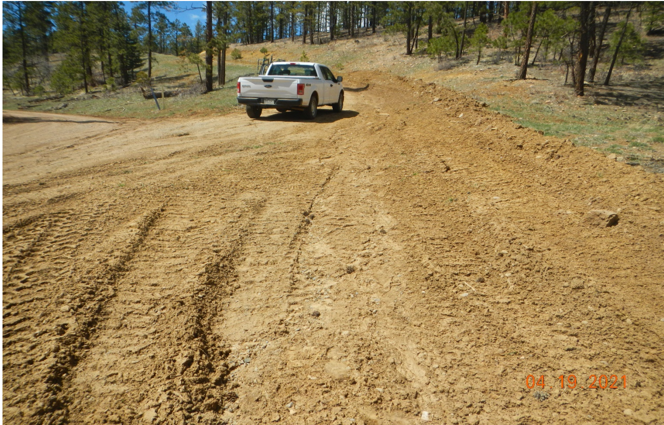
Photo 4. This graded disturbed area along the access road is susceptible to erosion and needs to be stabilized.
