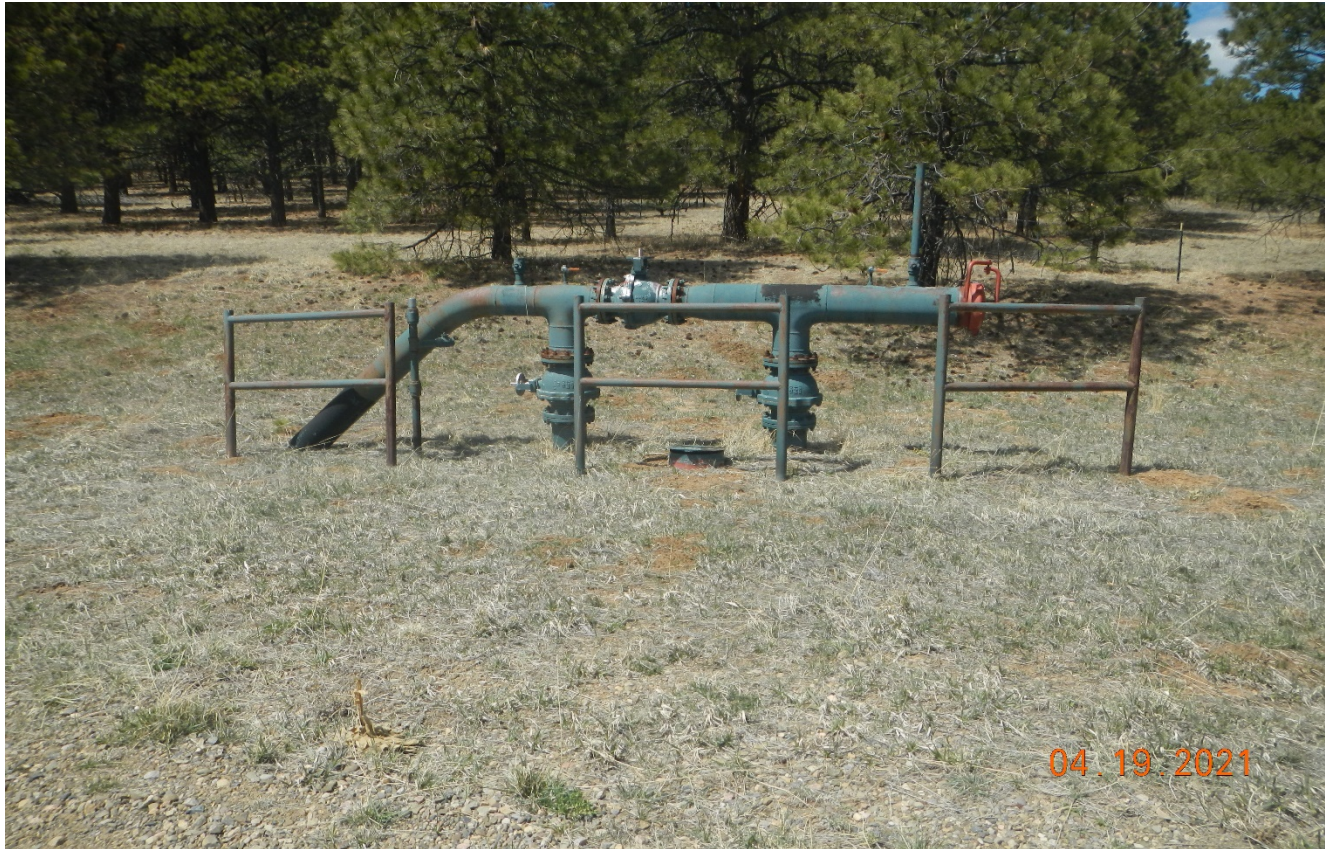
Photo 1. The pig launcher receiver remains along the access road which needs to be removed.
