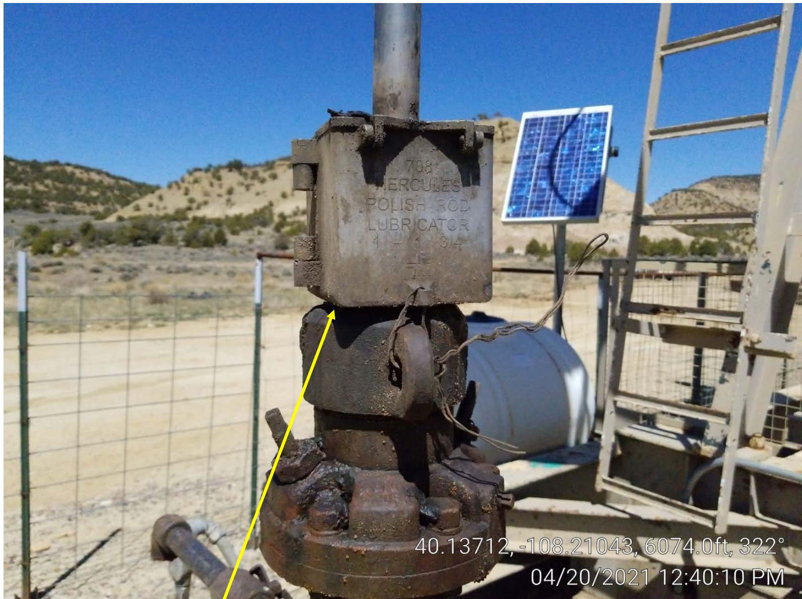
Photo 4. Gas leak at well.
