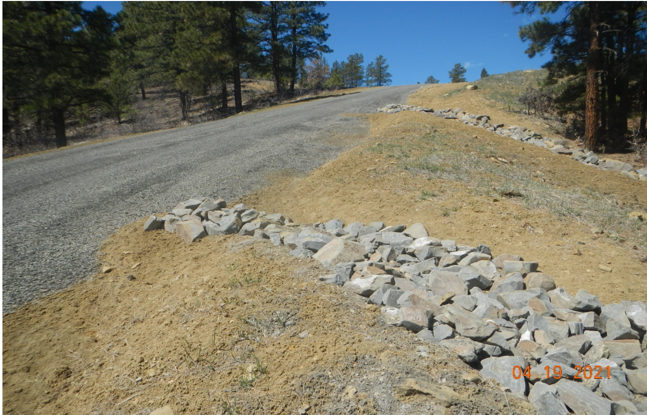
Photo 2. Rip/rap outlets were installed along the road near the location.
