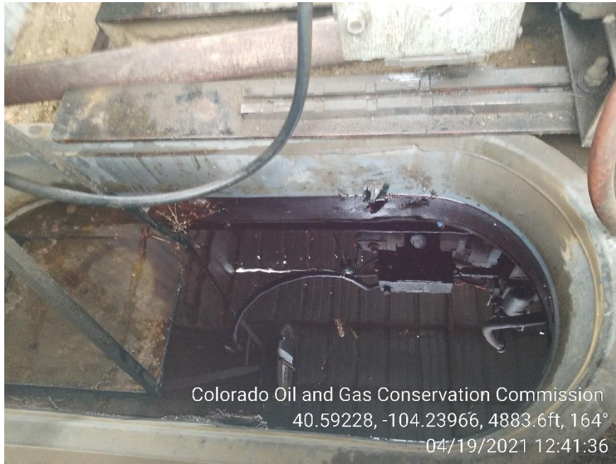
Photo 5 – Oily Waste in Secondary Containment
