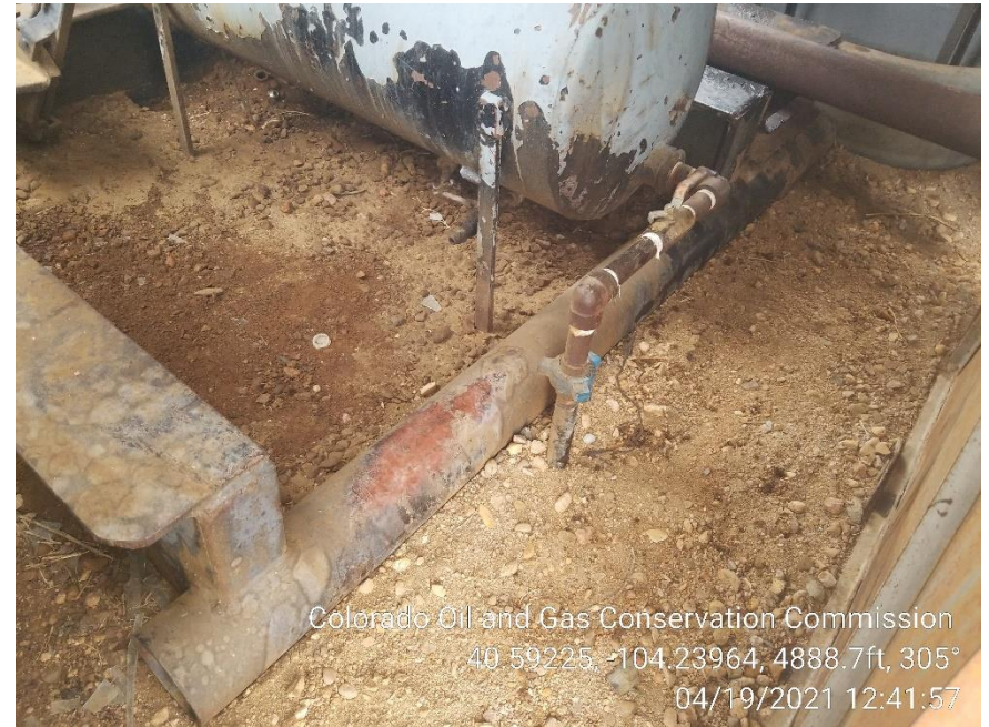
Photo 6 – Stained Soil at Gas Engine
