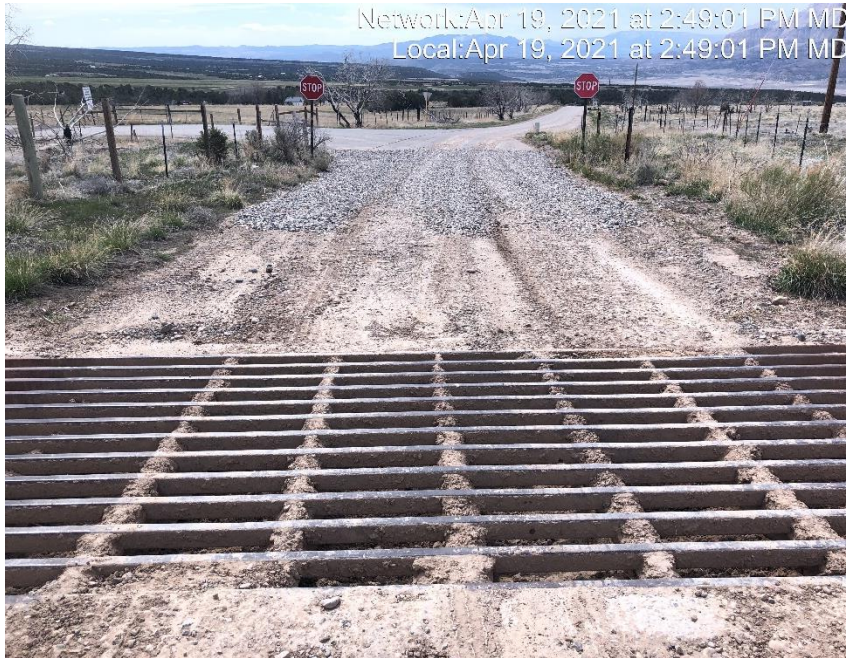
Photo #3551 Access road.
