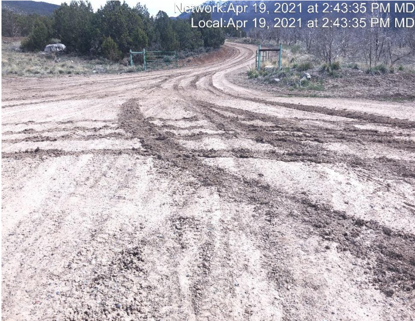
Photo #3550 No form of tracking BMP at entrance to location.
