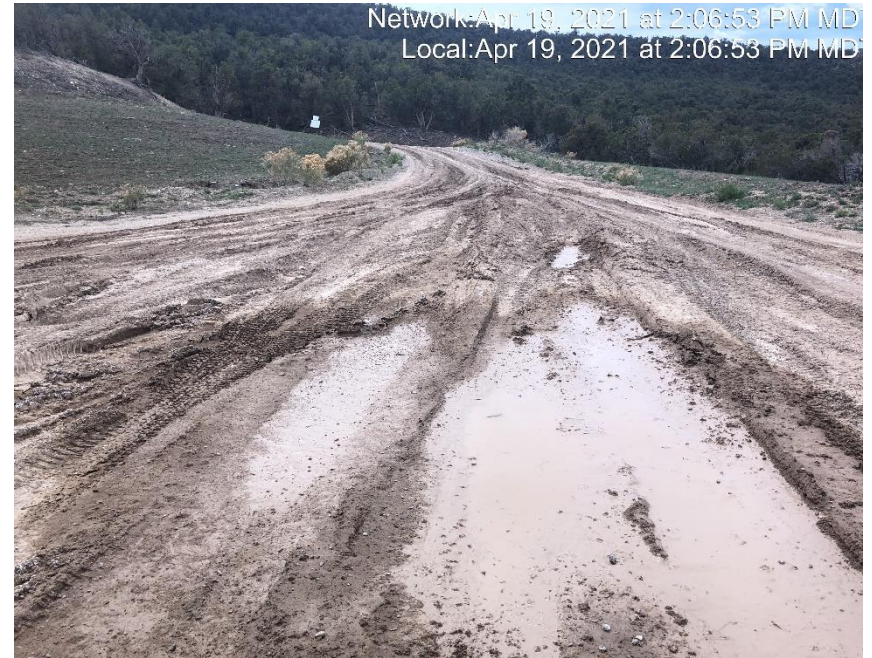
Photo #3542 No form of tracking control at entrance to location.
