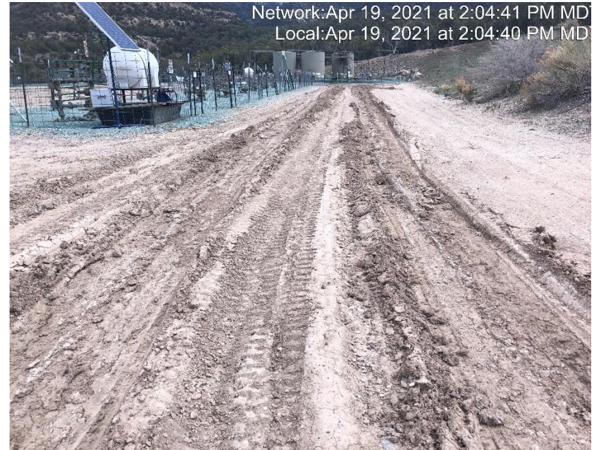
Photo #3540 Location lacks stabilization.
