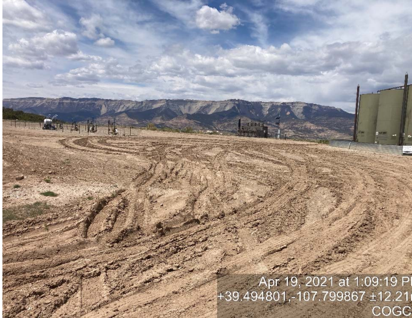
Location/lack of stabilization/compaction
