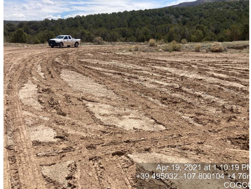
location/lack of stabilization/compaction
