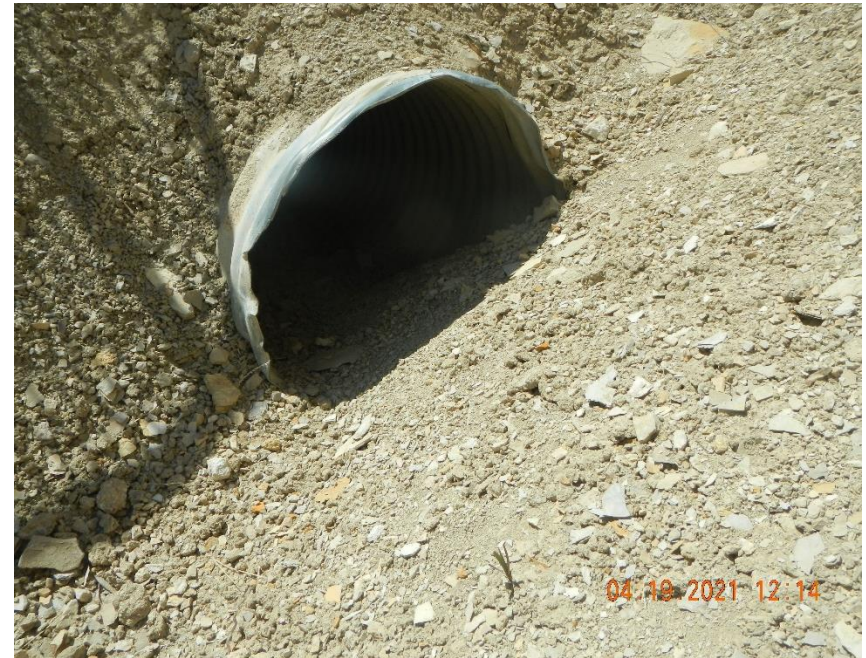
Sediment and shale in culvert basin and moving thru culver.
