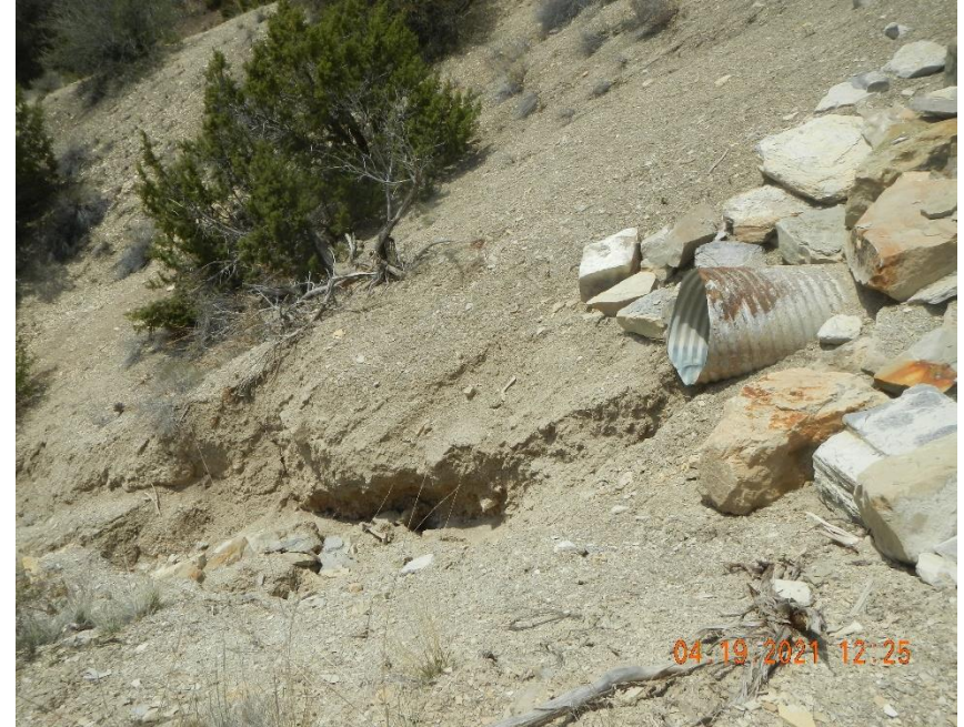
Flow from culvert creating erosion on outlet side of them.
