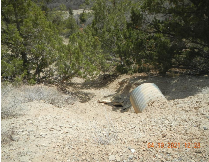
Flow from culvert creating erosion on outlet side of them.
