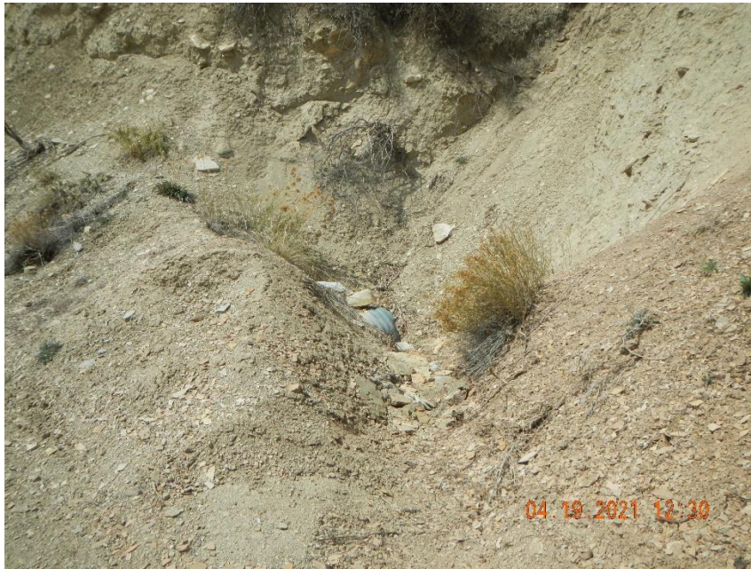
Sediment and shale in culvert basin and moving thru culver.
