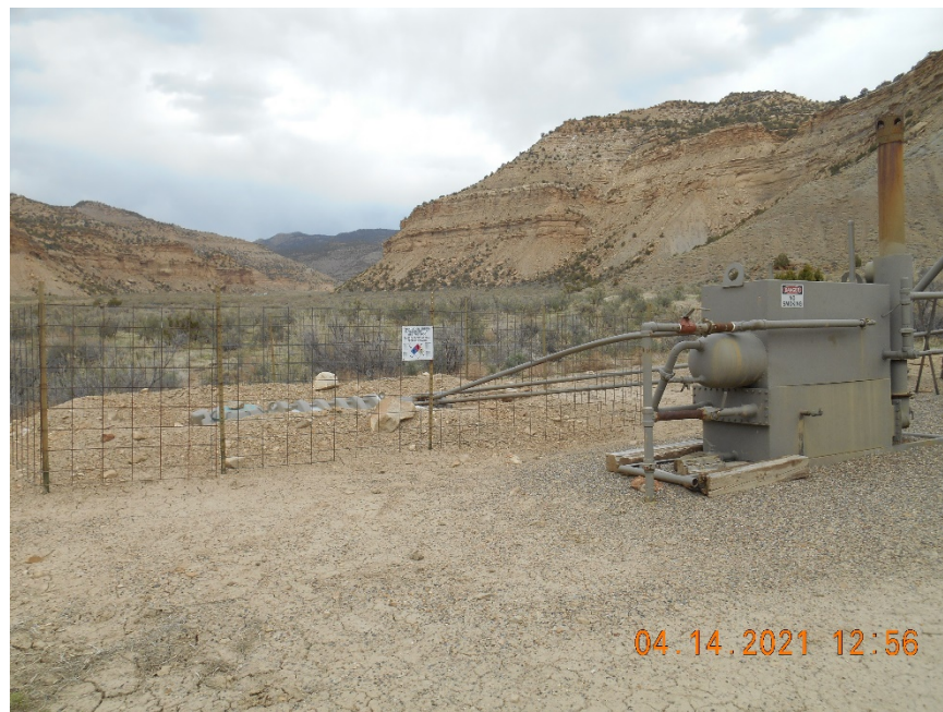
Separator and Tank battery with fence
