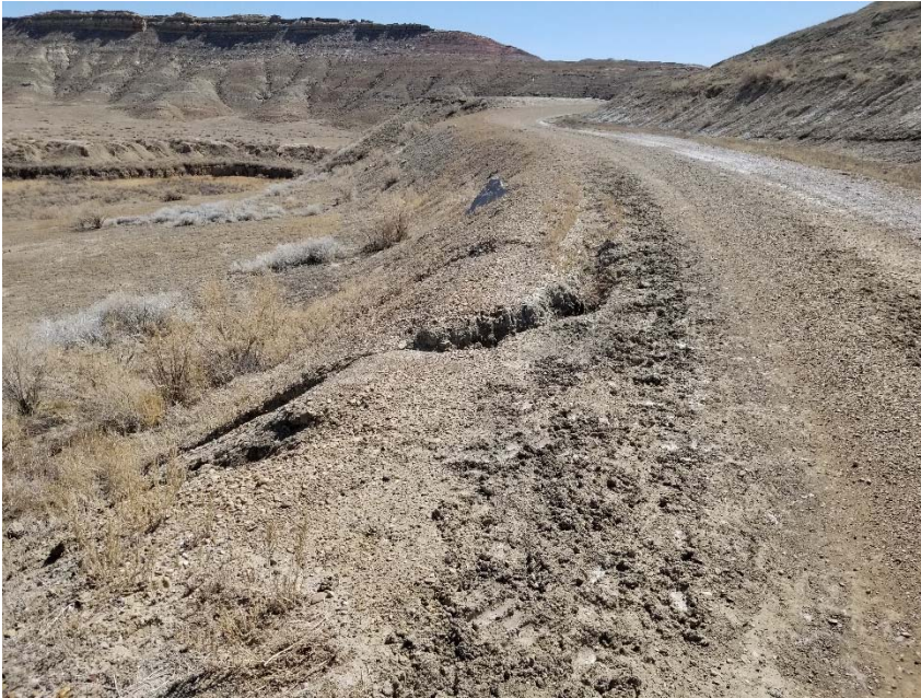
Photo 6. Erosion rill on access road.
