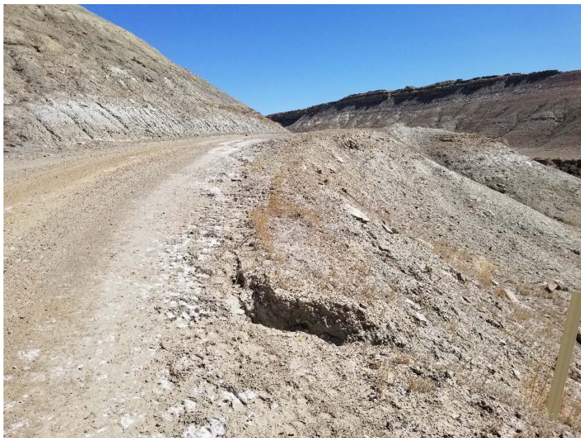
Photo 4. Erosion rill on access road.
