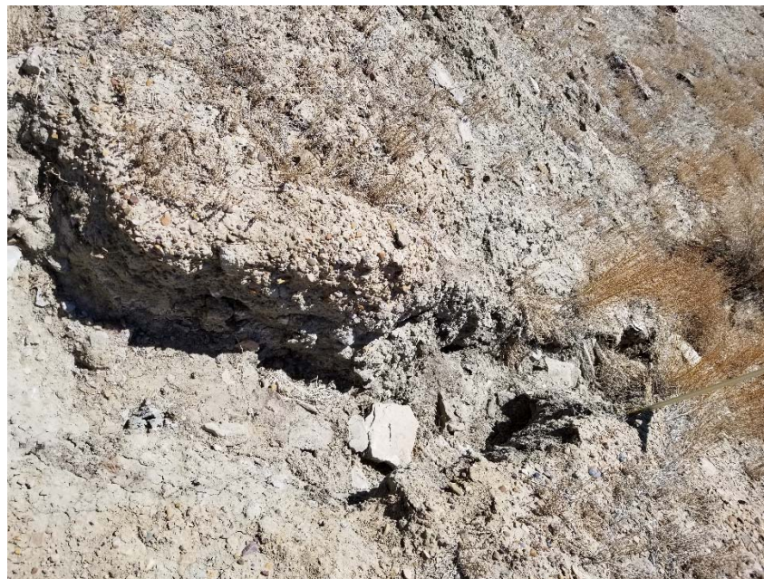
Photo 5. Sediment transport off access road.
