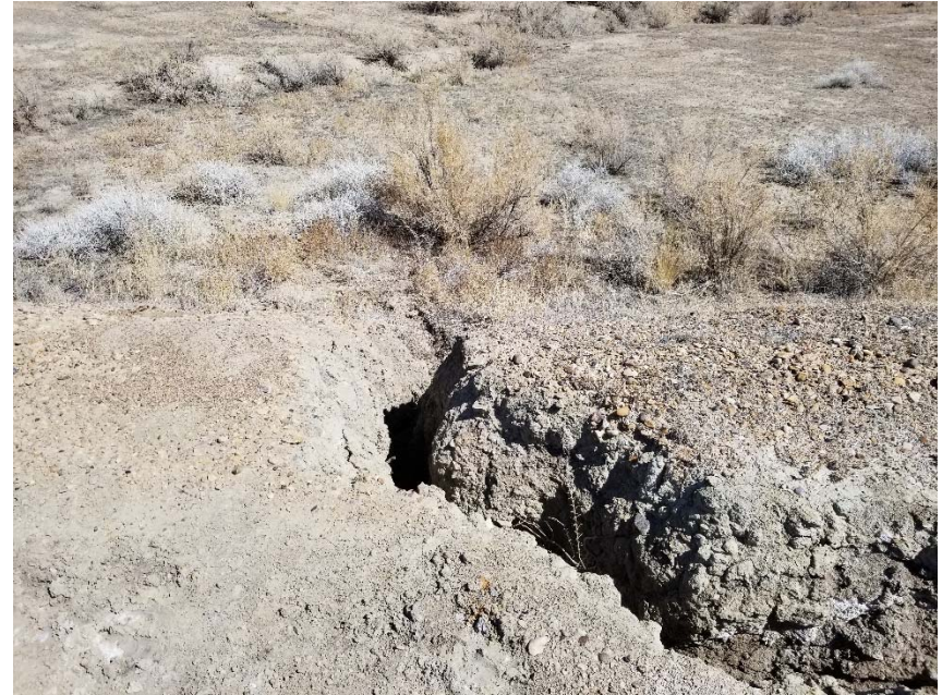
Photo 7. Sediment transport off access road.
