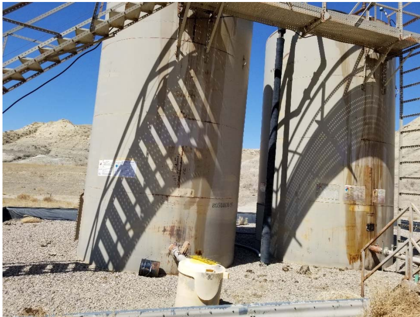
Photo 4. Tank labels faded/incomplete.
