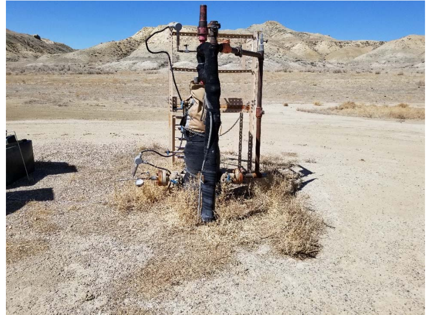
Photo 3. No bradenhead access apparent. Dried annual weeds on location.
