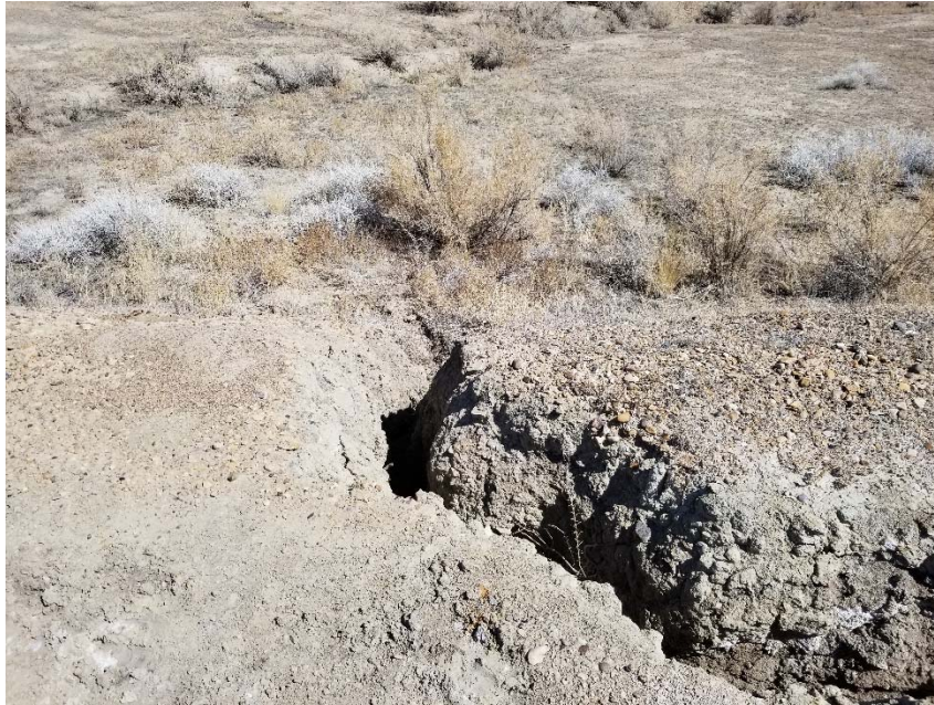
Photo 6. Erosion rill transporting sediment off access road.
