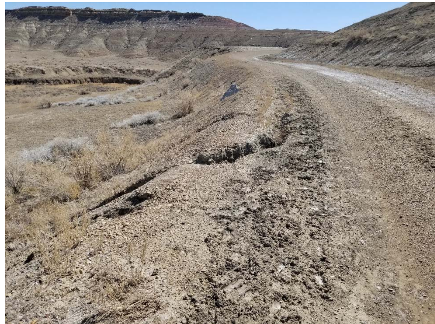
Photo 5. Erosion on access road.
