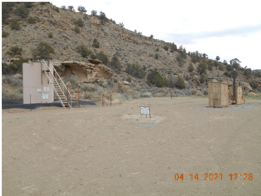
Location overview looking SE.
