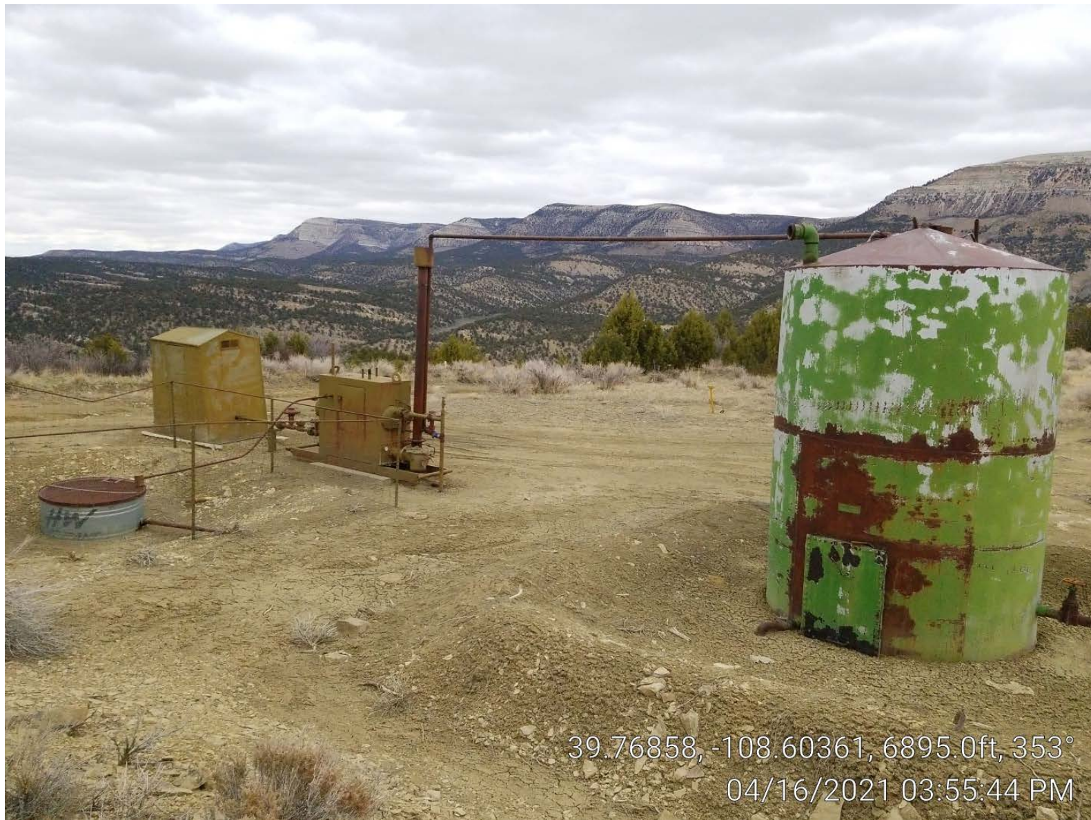
Photo 3. Tanks, meter building, separator.
