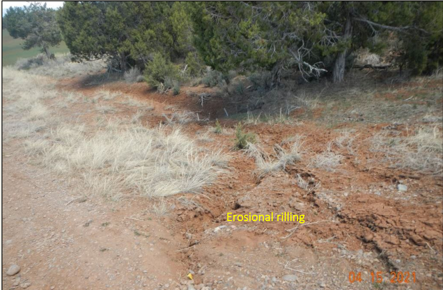
Photo 4. View of erosional rilling at the well pad entrance, facing downslope.
