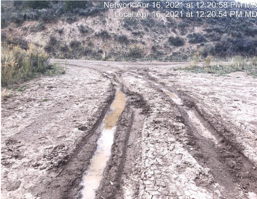
Photo #3511 no form of tracking control at entrance to location.
