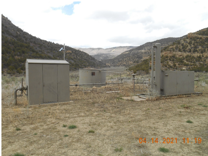
Meter housing, Produced Water tank and Separator.
