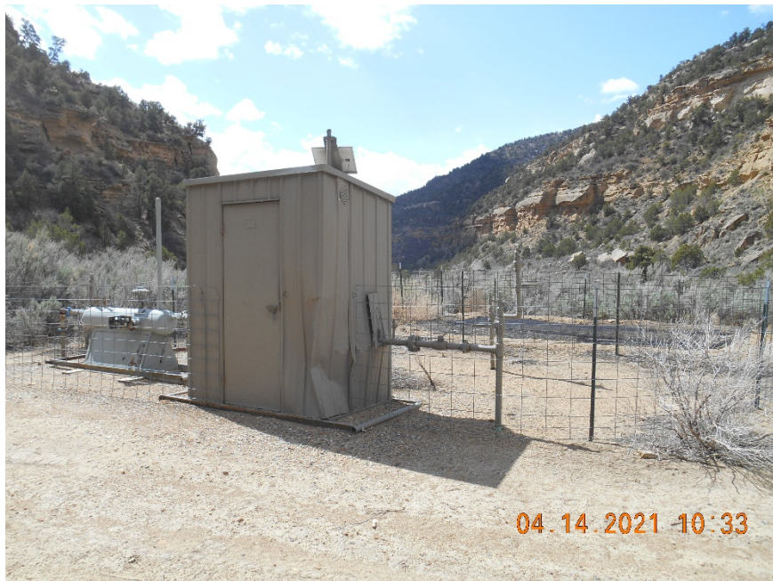
Separator and Meter housing (SE corner of pad)
