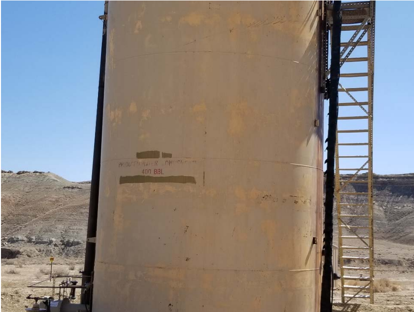
Photo 3. Tank label incomplete and faded.
