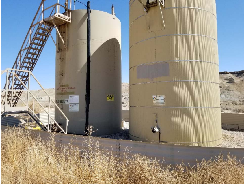
Photo 2. Tank labels faded or incomplete. Dried annual weeds.
