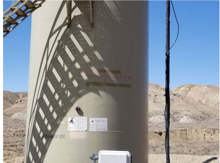
Photo 3. Incomplete/faded tank label.
