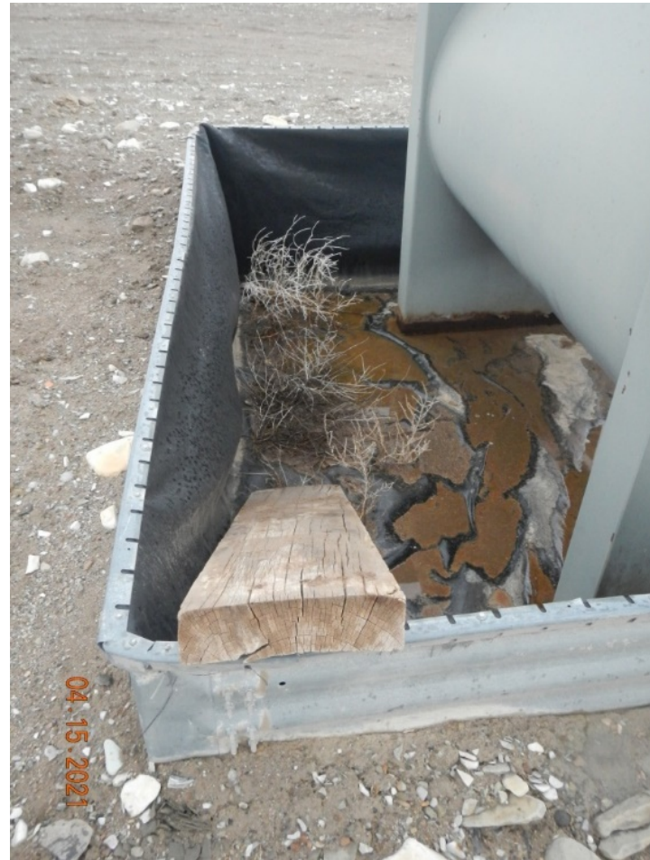
Photo#4: Escape board referenced in Inspection. Note Debris weeds blown into equipment.
