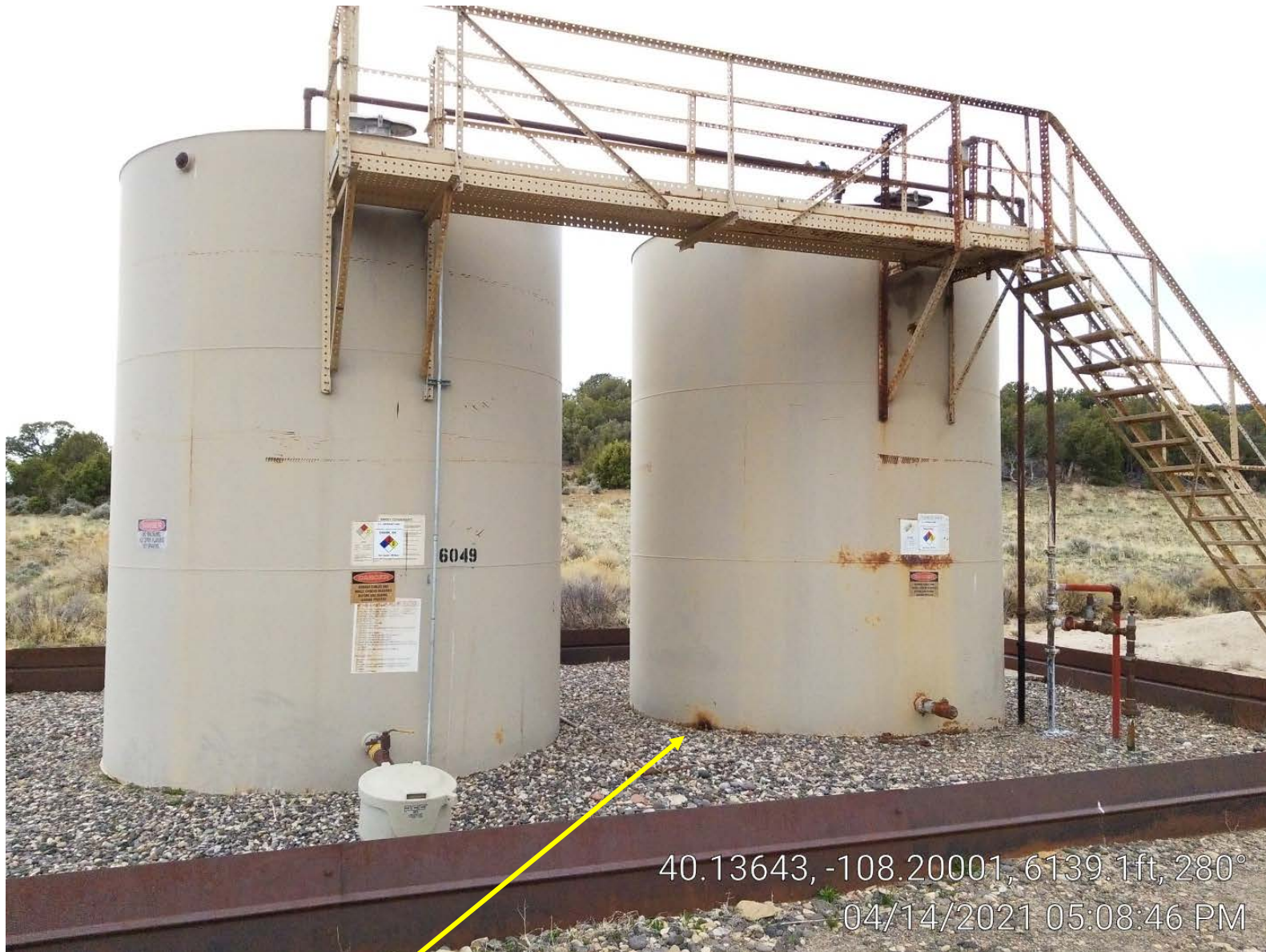
Photo 5. Tank with hole.
