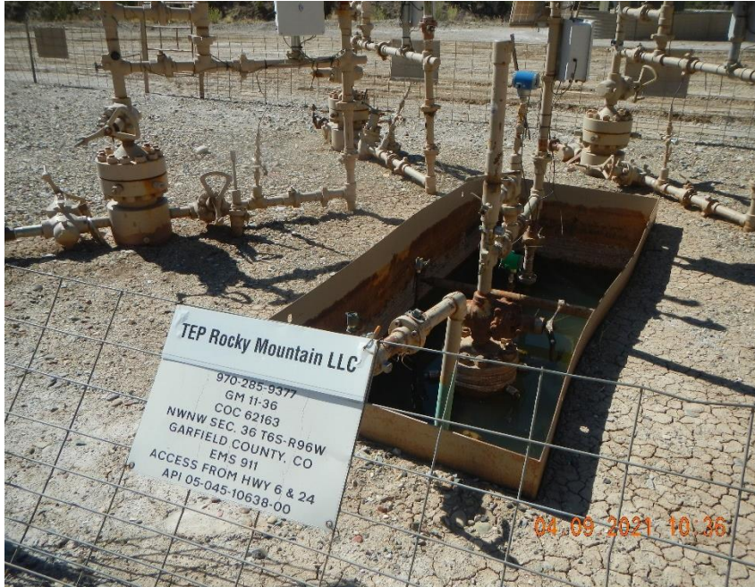
Storm water in metal well cellar.
