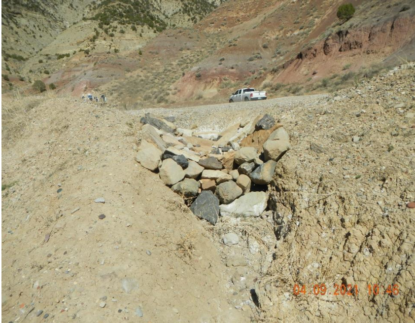
Erosion of drainage ditch and around rip rap.
