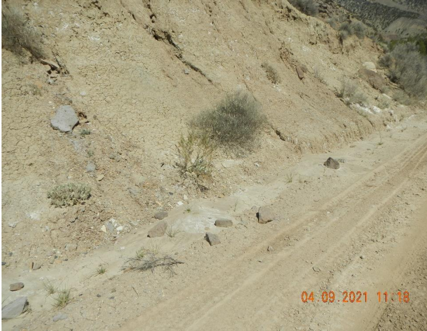
Sediment build up in ditch.
