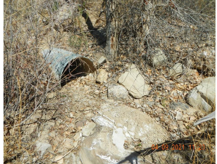
Sediment build up in culvert pipe.
