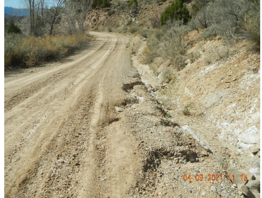
Erosion of road into the ditch.
