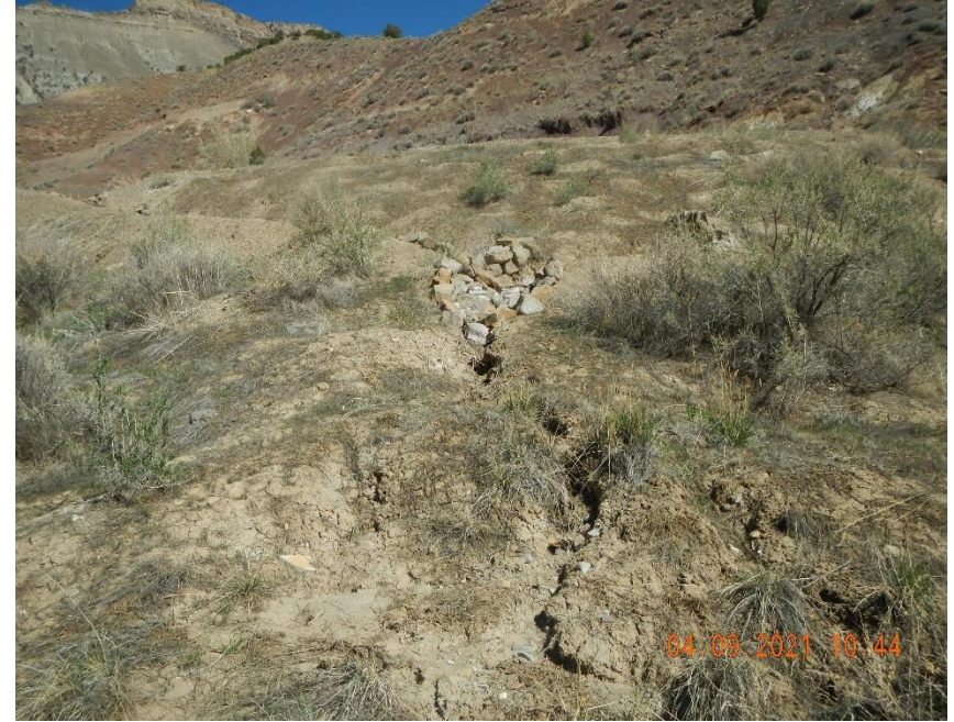
Erosion from check dam storm water flow.
