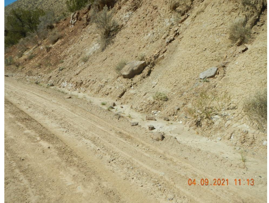
Sediment build up in ditch.
