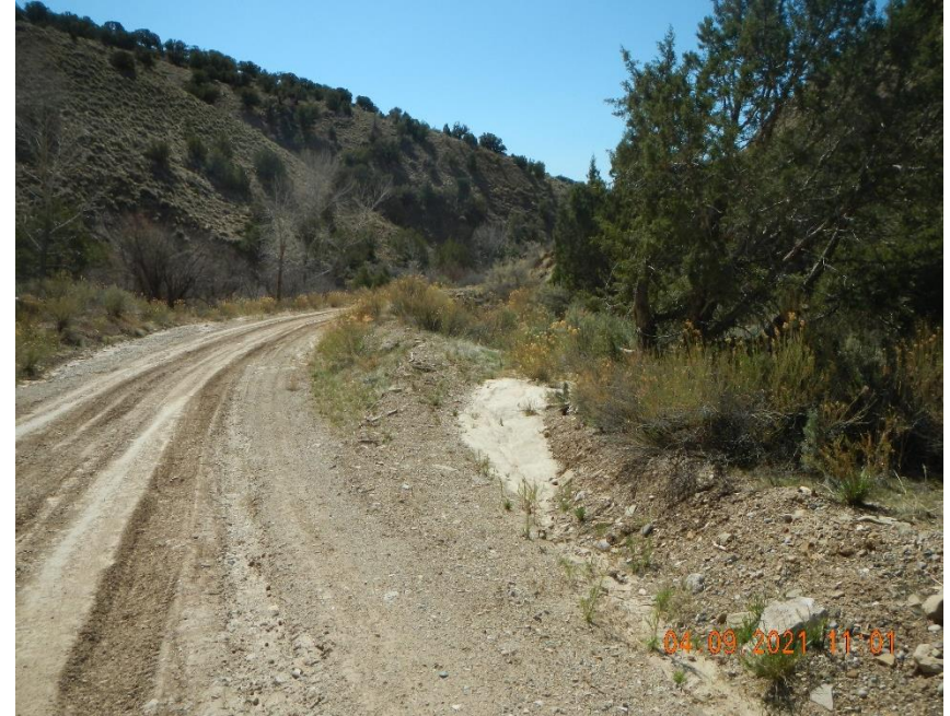
Sediment build up in ditch.
