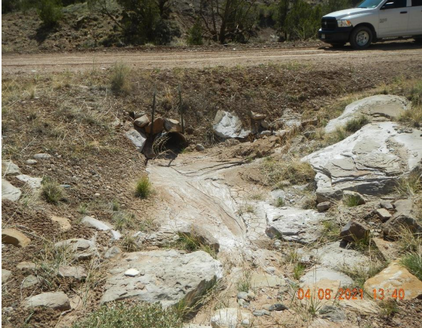
Sediment build up in culvert.
