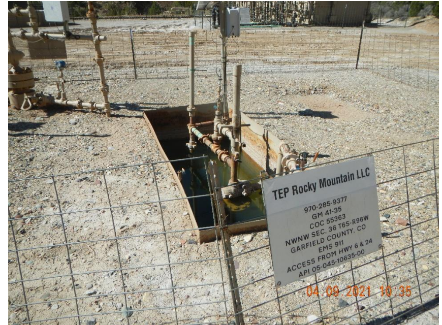
Storm water in metal well cellar.
