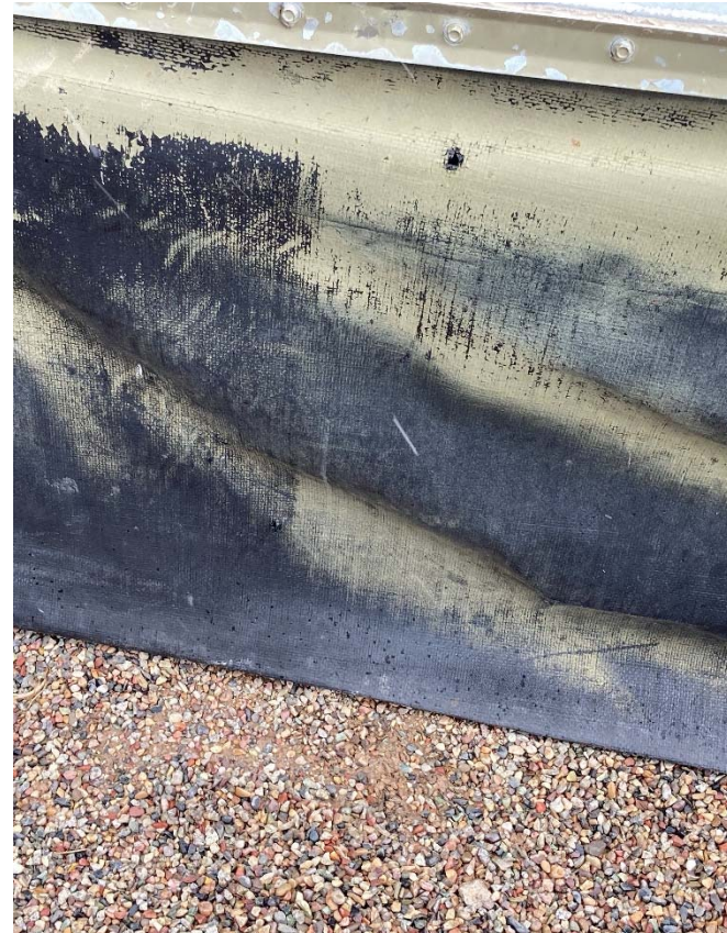
Multiple holes in containment
