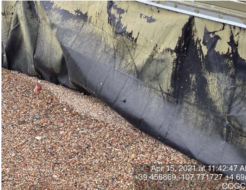
Multiple holes in containment
