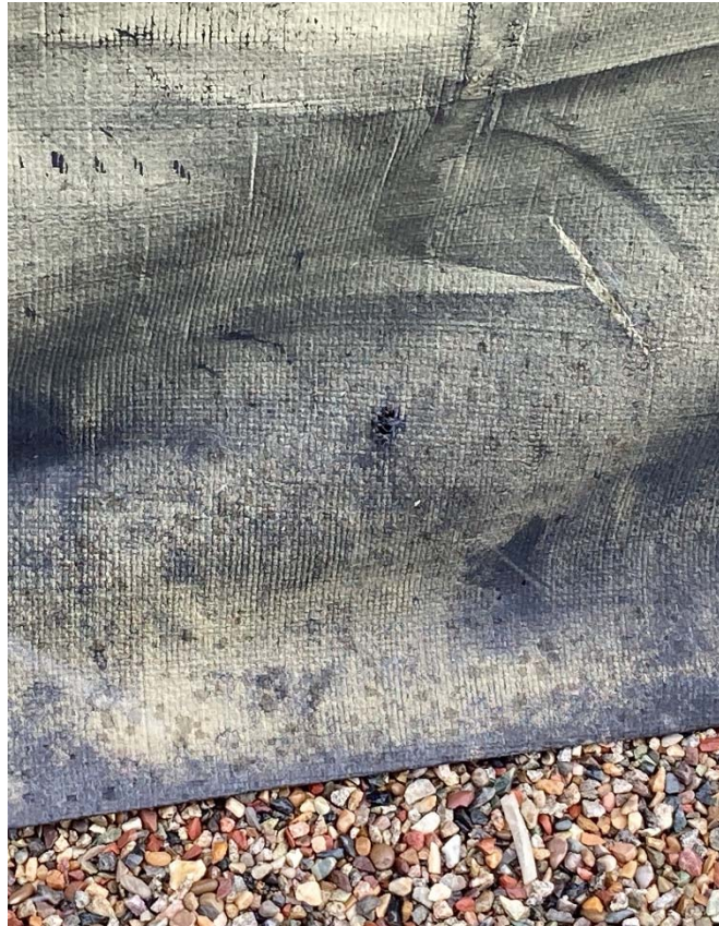
Multiple holes in containment
