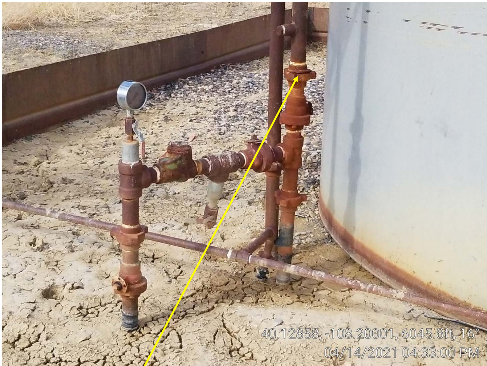
Photo 5. Cracked joint.
