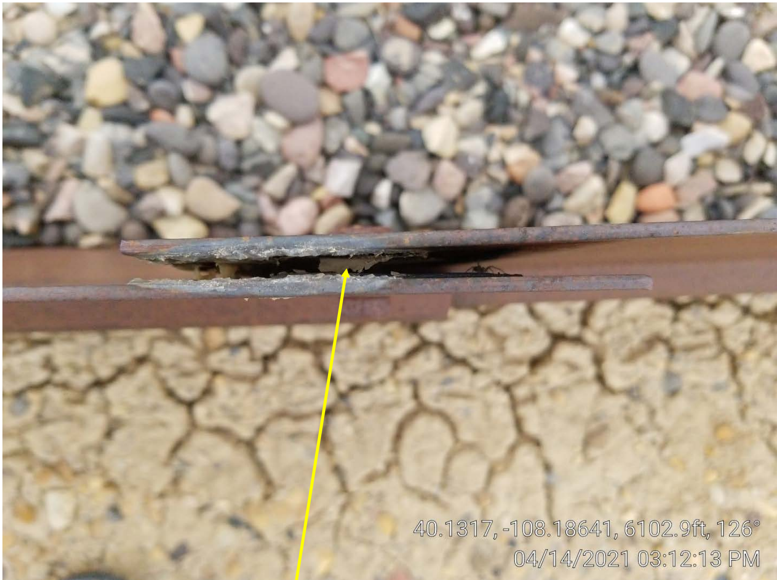
Photo 6. Gap in tank secondary containment.
