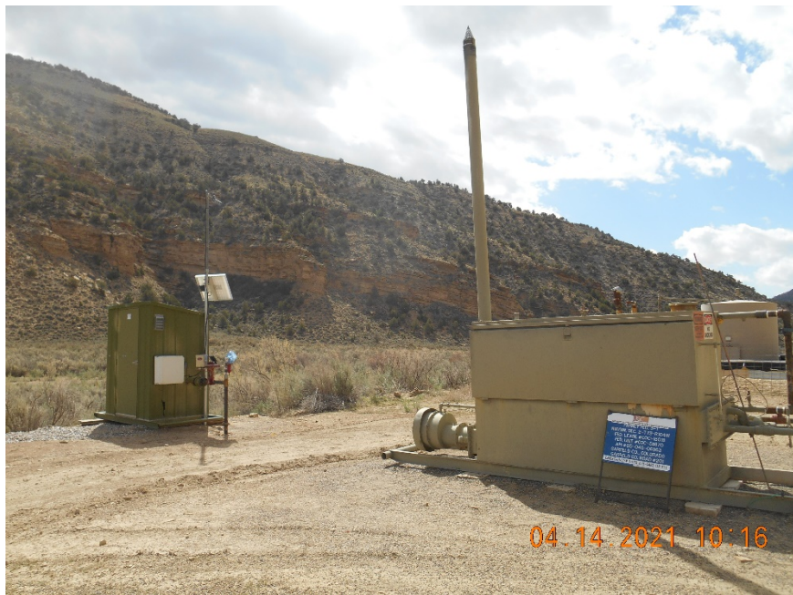
Separator and Meter Housing with sign
