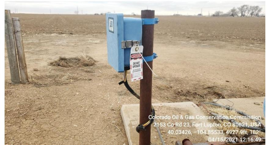
**Photo 4 WH Gas Engine start switch shut off and tagged out**
