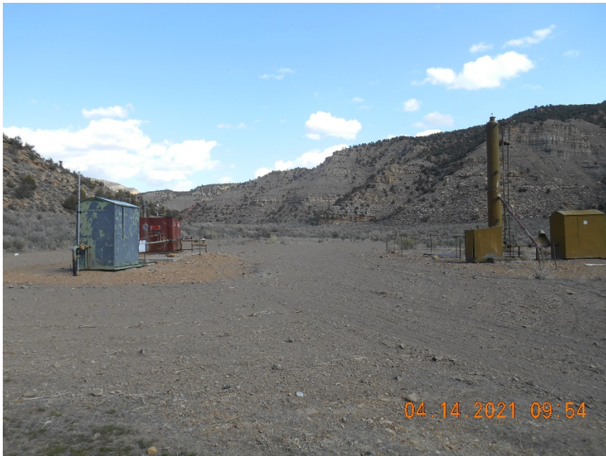
Location overview looking NE.
