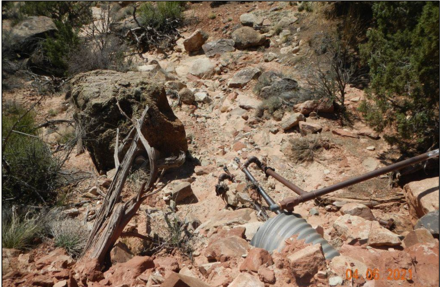
Photo 12. View of flowline at drainage intersection. Valve is open into drainage.
