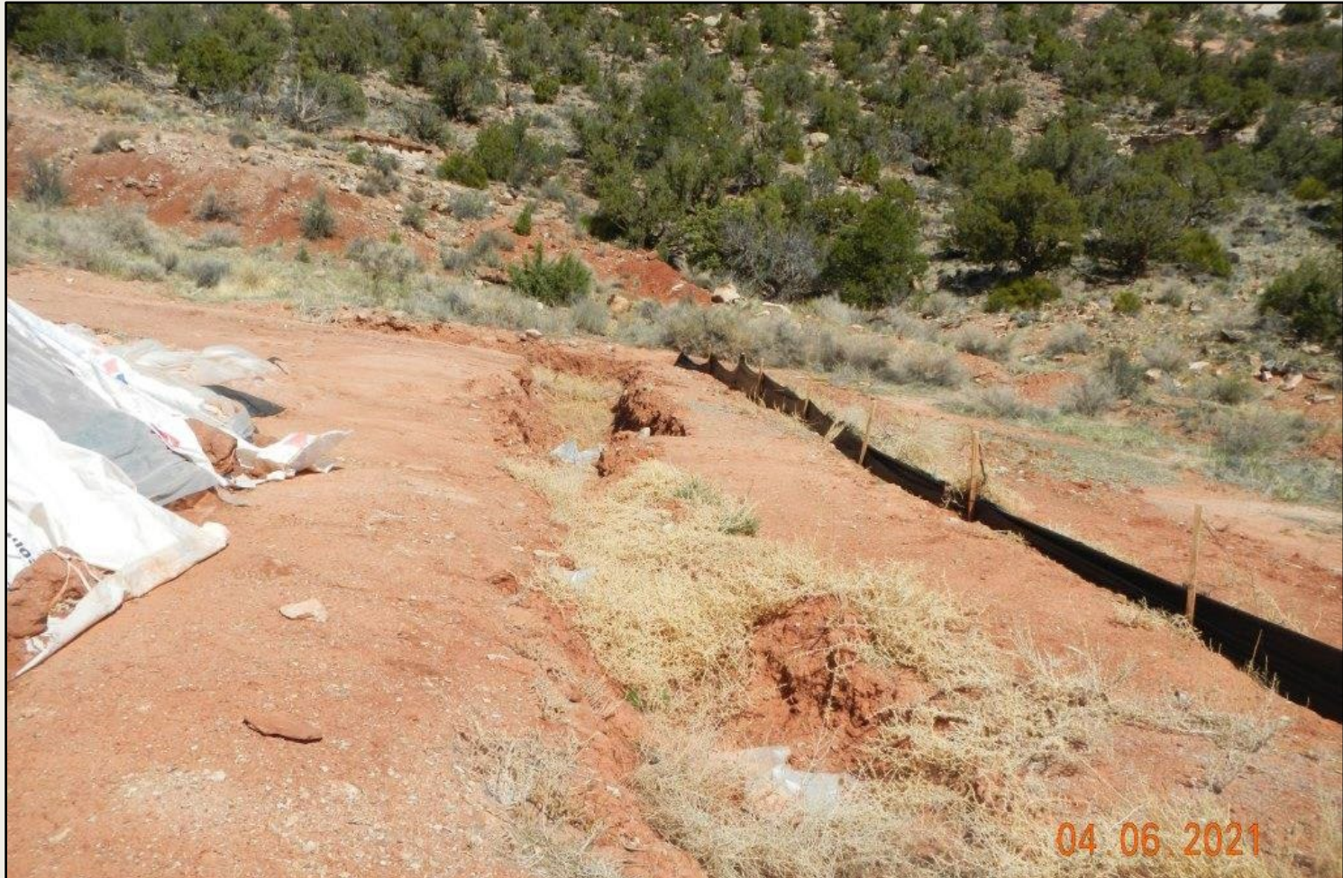
Photo 4. Another view of trench and silt fence in the eastern project area. Russian thistle and plastic debris observed in trench.
