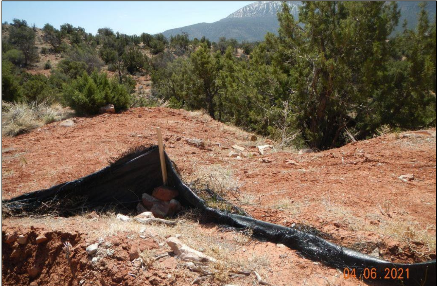
Photo 3. View of silt fence in the southeastern project area, in disrepair.
