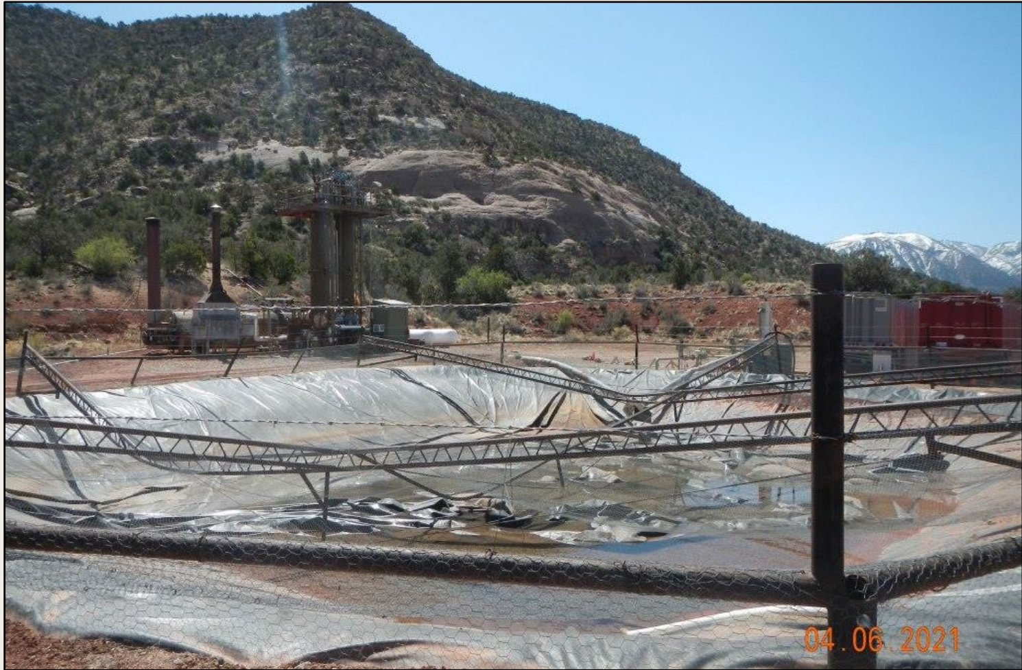
Photo 2. View of the project area from the northwestern corner facing center. Netting scaffold appears to have collapsed. Netting in disrepair.
