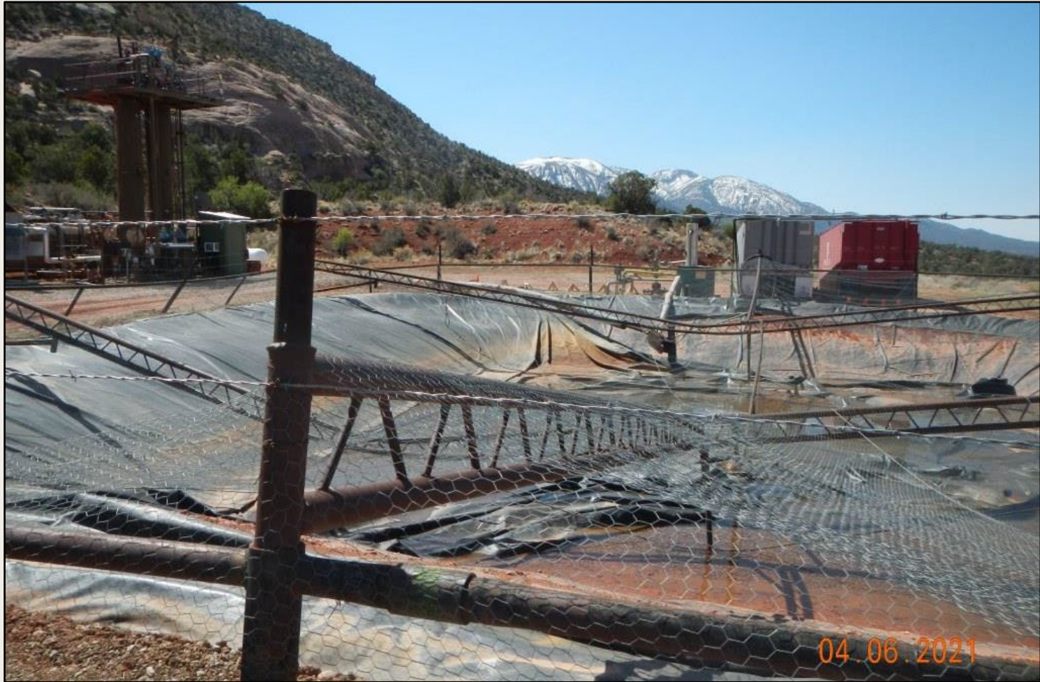
Photo 3. Another view of pit area. Liner may be compromised. Netting in disrepair.
