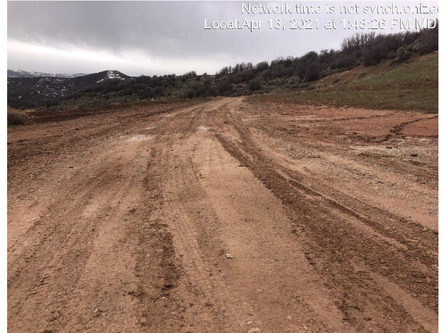
Photo #3474 No form of tracking control at entrance to location.
