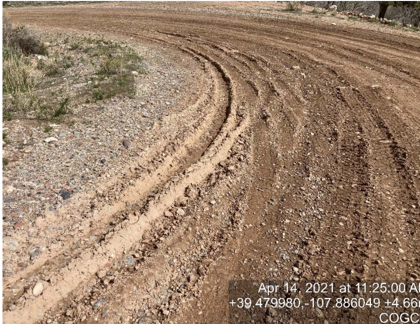
Lack of stabilization/compaction
