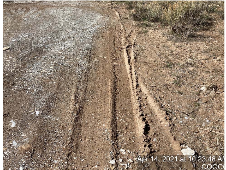
Lack of stabilization/compaction
