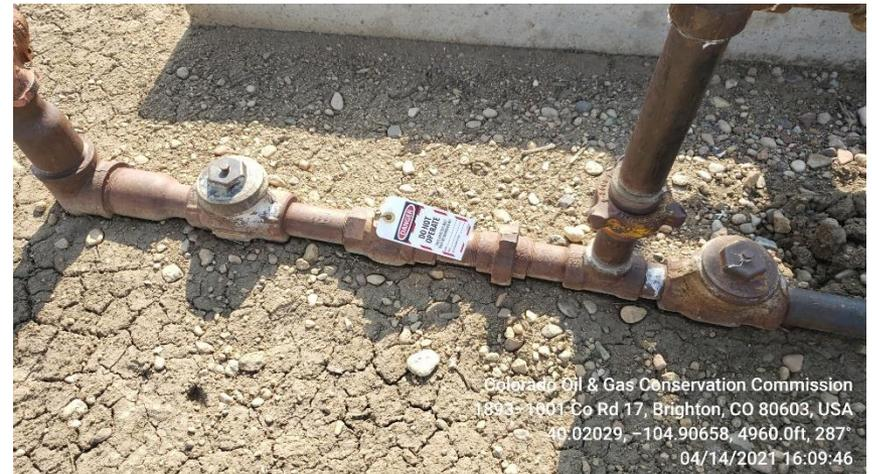
Photo 3 Valve closed and tagged out
