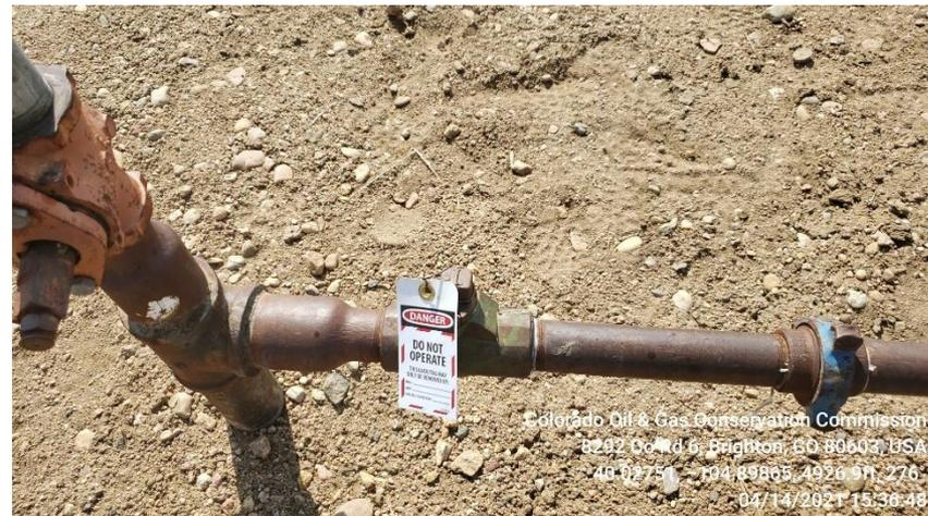
Photo 3 Valve closed and tagged out
