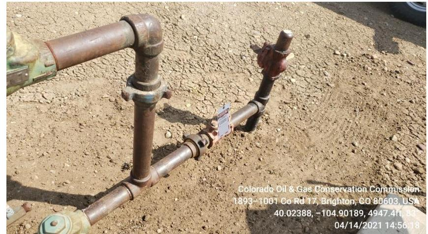
**Photo 3 Valve closed and tagged out**
