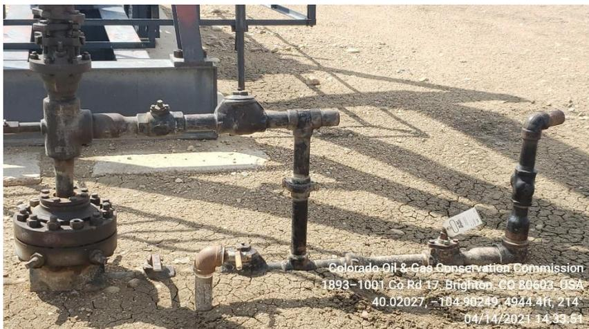
**Photo 3 Valve closed and tagged out**
